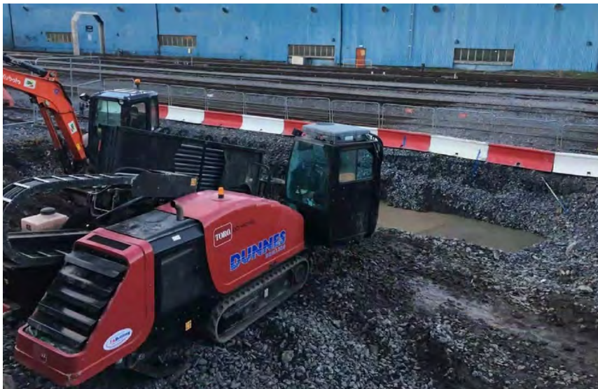
Image 5-4 Directional drilling plant, in position (Source: IÉ)
