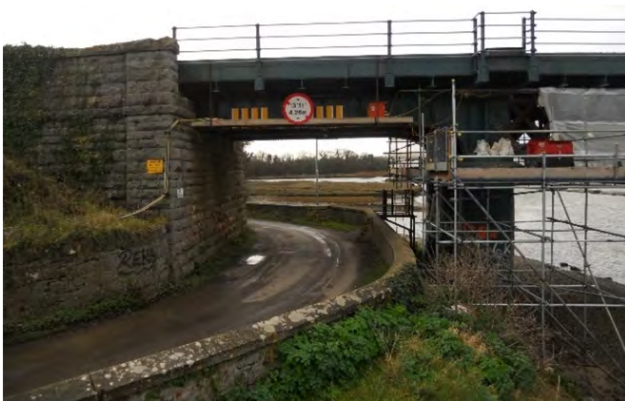
Image 5-102 Example of previous scaffolding access (Source: IÉ)
